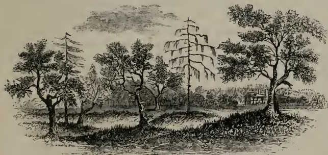
VIEW OF THE REMAINS OF THE FRENCH WORKS. a
